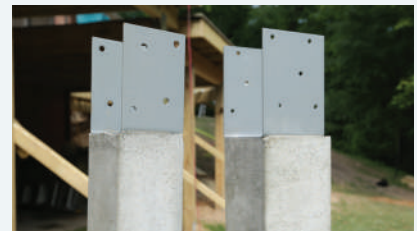
PRECAST CONCRETE DECK POSTS
