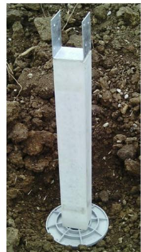
Figure 8.1: Deck Post on Molded Composite FootingPad
